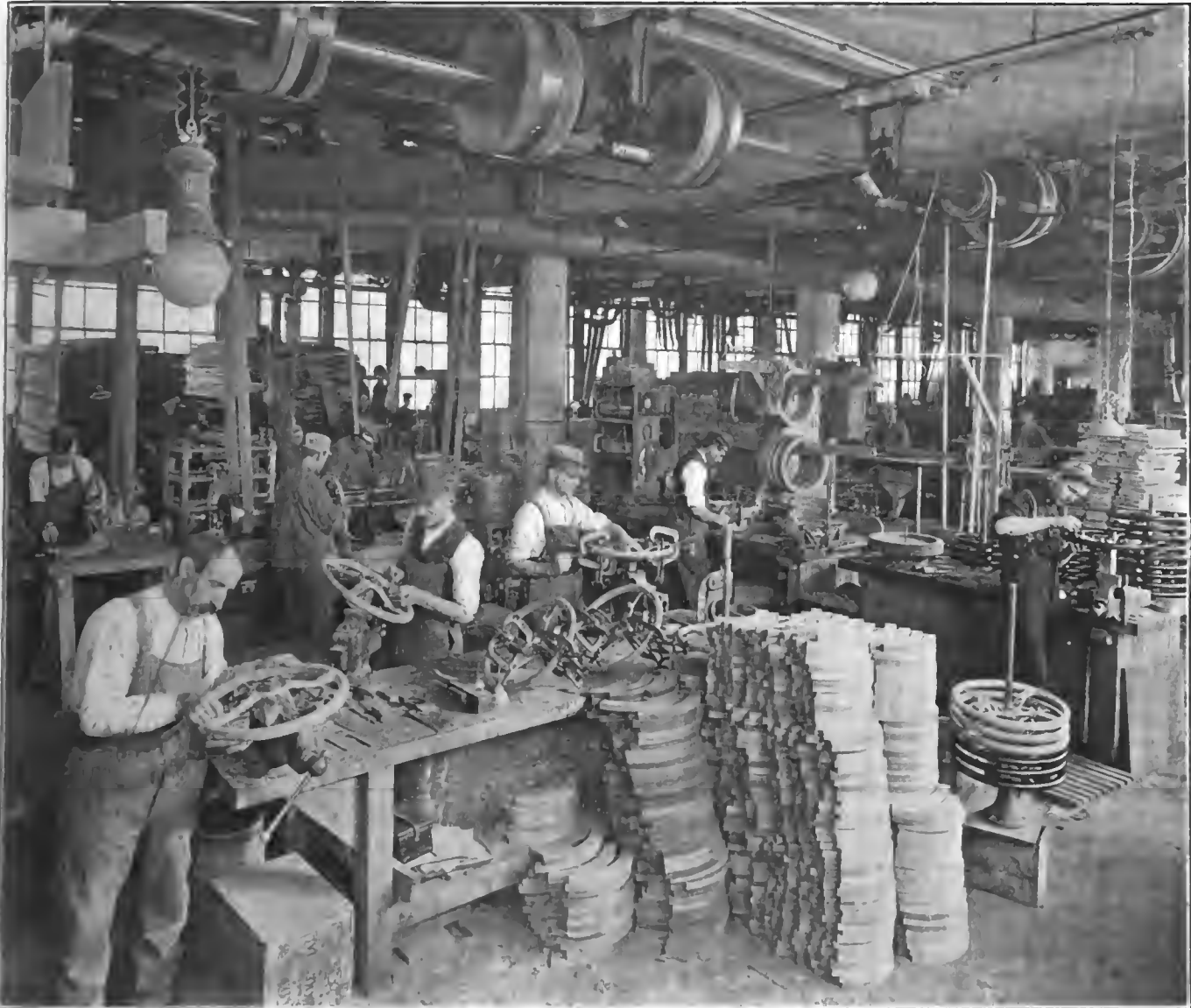
SHOWING PROCESSES IN THE MANUFACTURE OF MAHOGANY RIMS FOR STEERING WHEELS—PACKARD
